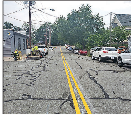
Figure 1: Final Product - Crack Sealed Roadway
