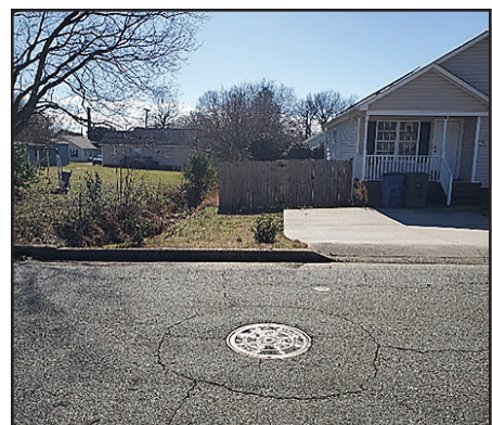
Figure 5: Transverse/Block Cracking
