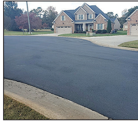
Figure 3: Final Product - Resurfaced Roadway
